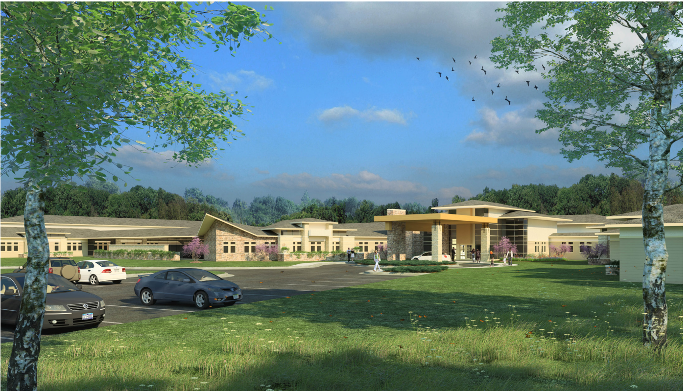
Architect's rendering of the facility prior to construction. Image credit: Wendel (formerly ADG)
