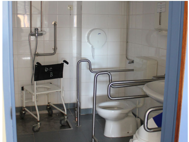
Figure 49 Hospital Curry Cabral (PT) Toilet
