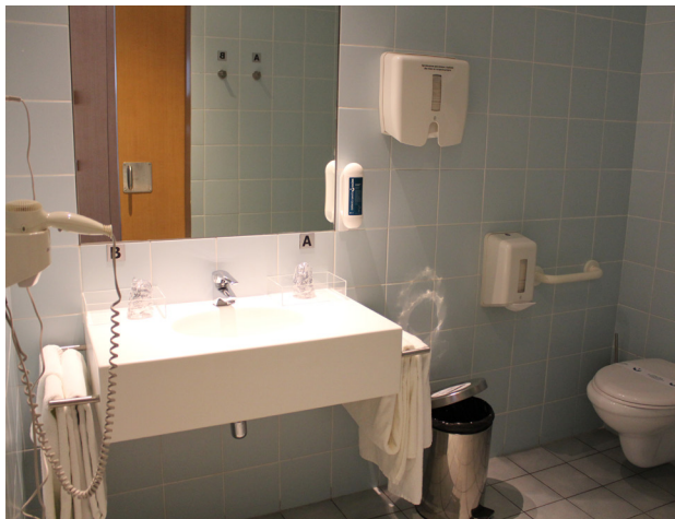
Figure 30 Hospital da Luz (PT) - Toilet (from double room)
