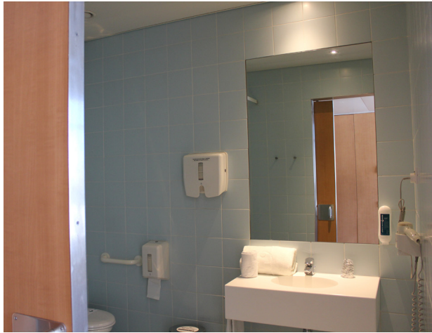
Figure 28 Hospital da Luz (PT) - Toilet
