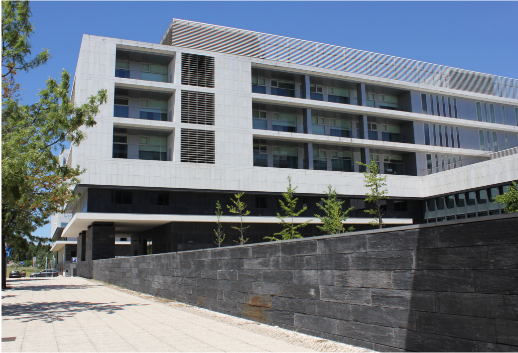
Figure 21 Hospital da Luz (PT) - exterior
