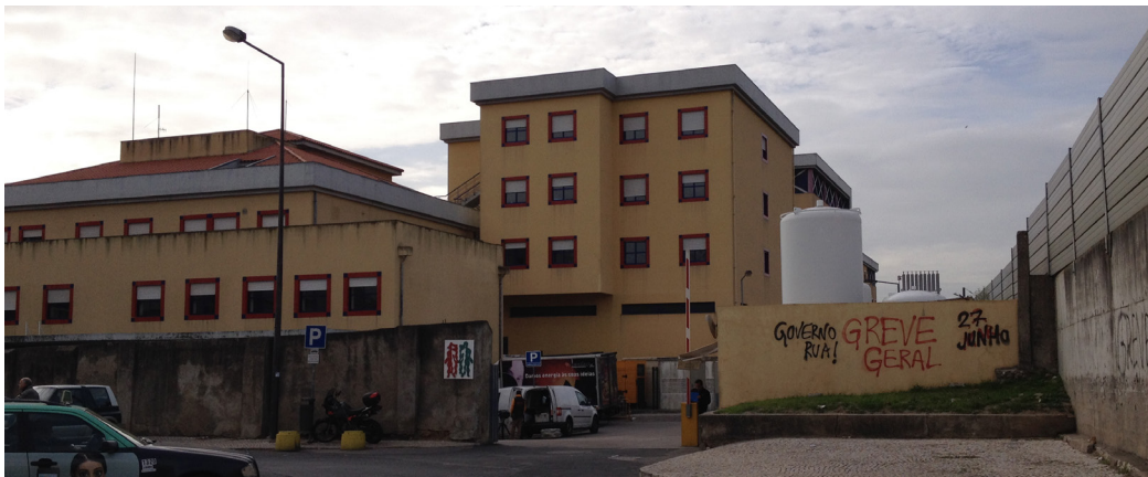
Figure 43 Hospital Curry Cabral (PT) - exterior
