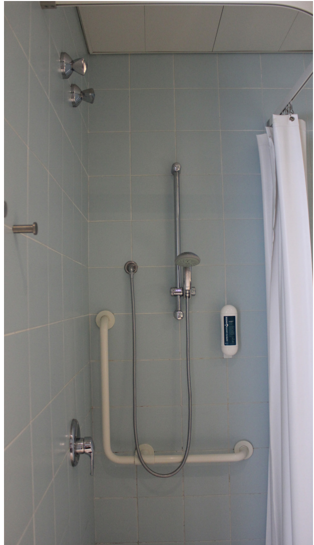
Figure 29 Hospital da Luz (PT) - Toilet
