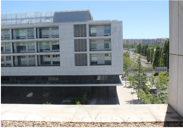
Figure 31 Hospital da Luz (PT) - View 1
