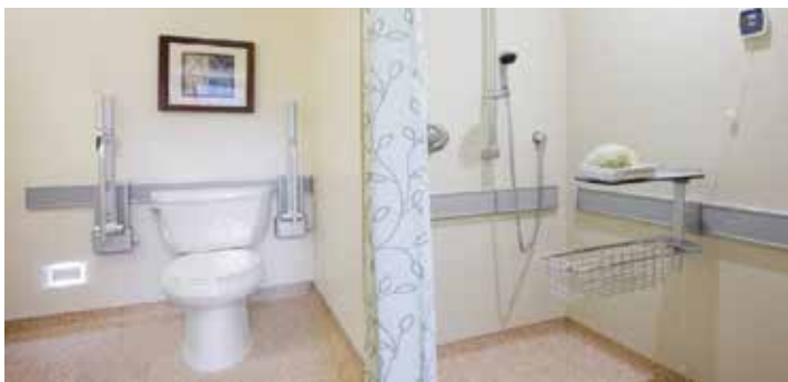
PICTURE 8 Bathroom with grab-bars on both sides of toilet New Bridge on the Charles (long-term care setting)
