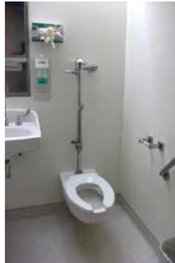
PICTURE 6 Bathroom with single diagonal grab-bar at the toilet
