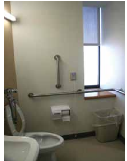
PICTURE 7 Bathroom with grab-bars on multiple walls Paoli Patient Care Pavilion
