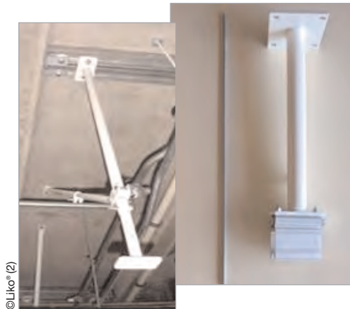
Figure K-10: Pendant Attachment
