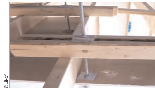
Figure K-11: Threaded Rod Mount
