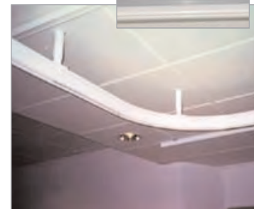
Figure K-7: Suspended Track
