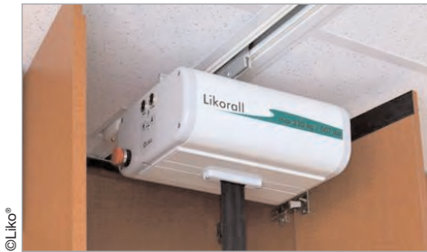
Figure K-8: Recessed Track
