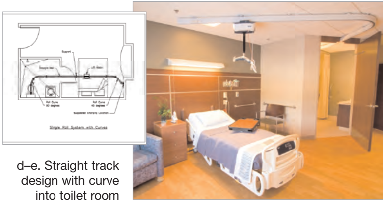
K-5: Ceiling-Lift Tracks Extending from Patient Room into Toilet Room
