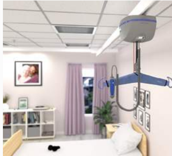
Arjo Ceiling-mounted lift in a resident room
