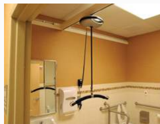
Ergolet Wall-mounted overhead lift in bathroom
