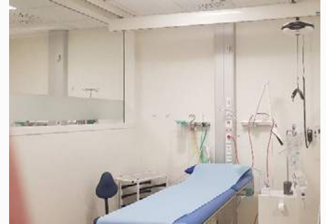
Ergolet Ceiling-mounted lift in an emergency department
