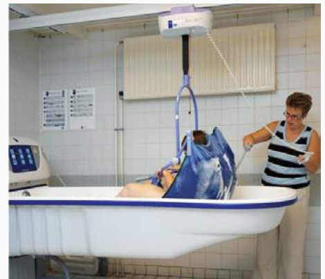
Arjo Ceiling-mounted lift in a bathing room
